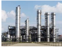
Oil and gas pipeline surveillance
